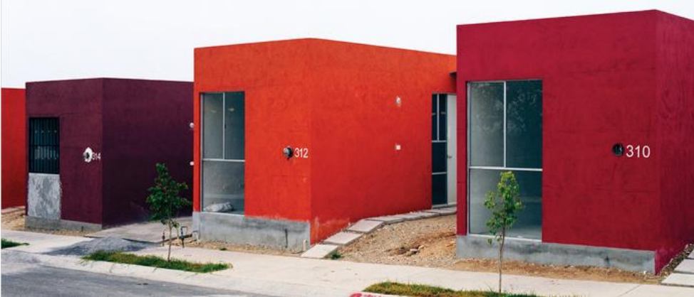
Suburbia Mexicana by Alejandro Cartagena in Toronto's Warden Subway Station, Contacting Toronto, 2015
